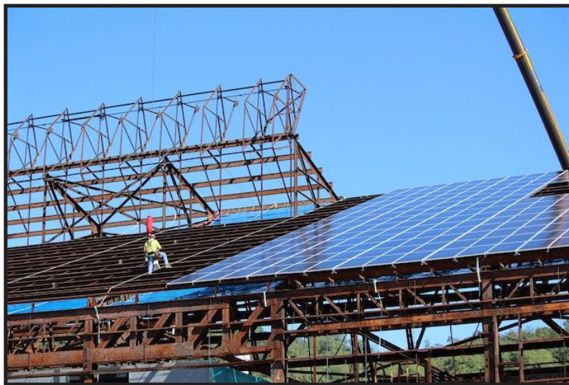
Solar work in progress. Photo courtesy of Scalo Solar Solutions
