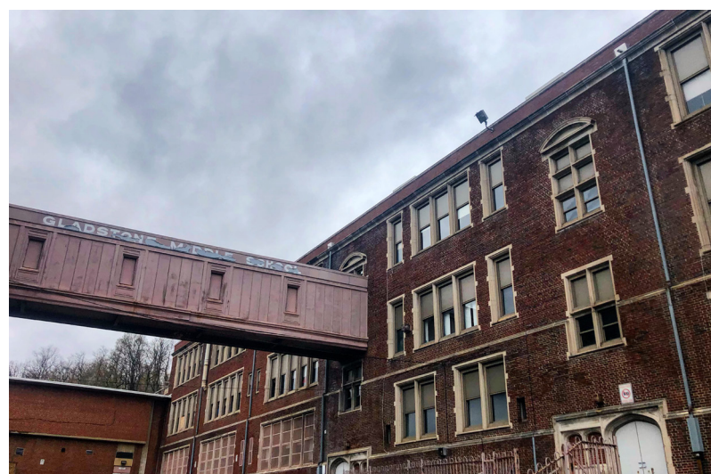
The main Gladstone Middle School building which is to become affordable rental housing units.
